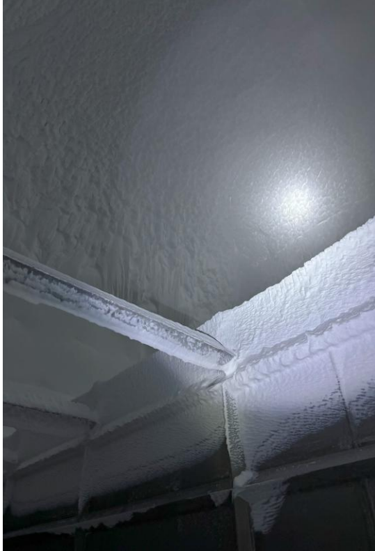
Extensive dust at granulator ceilings and stiffeners
