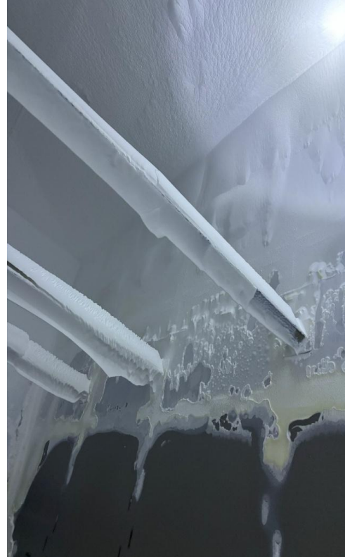
Extensive dust at granulator ceilings and stiffeners
